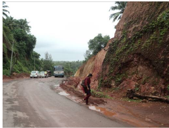
Plate 7.1. Major cut section inlink no. 69, which will be further widened as a part of the project
