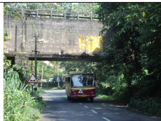
Figure 7.4. Project road Crosses an aquaduct at km 47+560 at Uthimoodu
