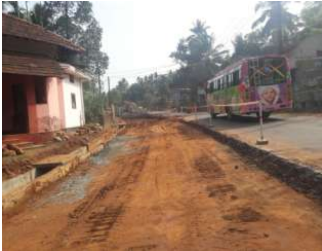
EXCAVATION UPTO SUBGRADE WORK IN PROGRESS AT KM.4+700
