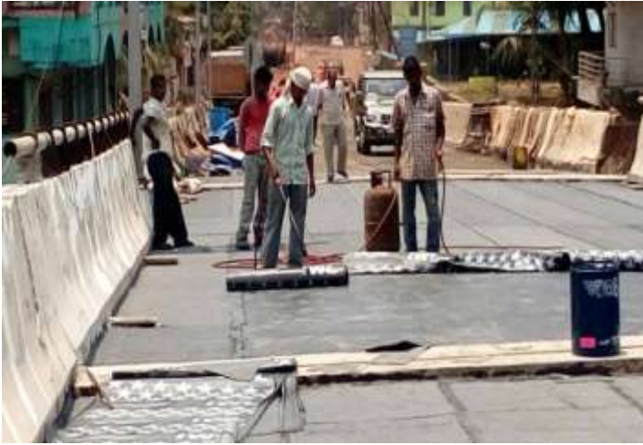
HYPER PLAST POLY MEMBRANE FIXING OVER PAPPINISSERY ROB (KM 19+950)
