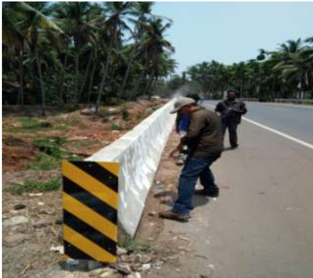
CONCRETE SURFACE GRINDING AT KM 6+520 (LHS)
