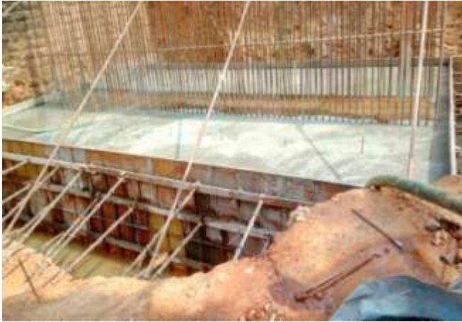
ABUTMENT A2 PILE CAP OF MAJOR BRIDGE AT KM 42+195
