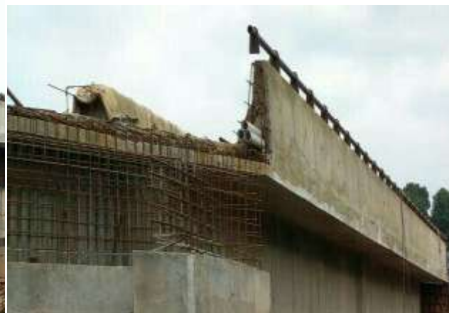
PROVIDING HAND RAIL FOR MINOR BRIDGE CRASH BARRIER (CH: 0+380 KM)
