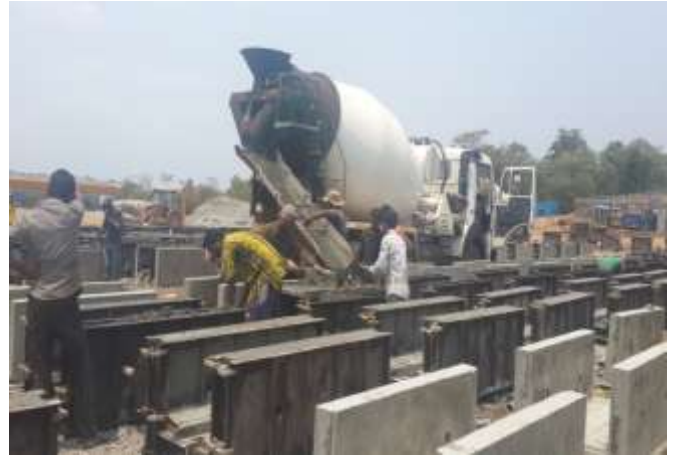
PRE CAST DRAIN CONCRETE AT CASTING YARD
