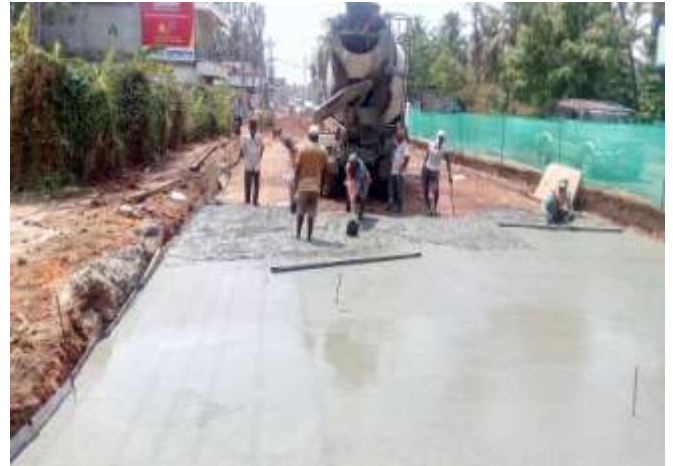
BOX CELL PCC WORK IN PROGRESS ON A2 APPROACH OF THAVAM ROB (KM 7+420)
