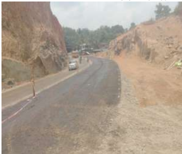
PRIMING COMPLETED @ CH 30+400 TO KM 30+520
