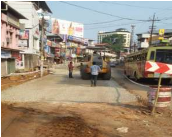
WMM COMPLETED AT CH. 16+480 TO 16+600 (LHS)
