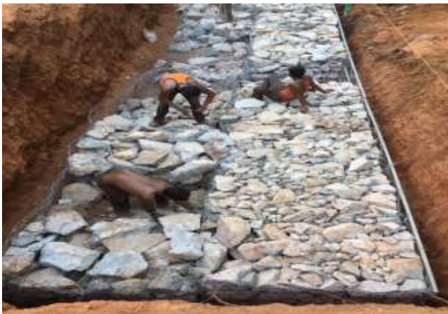
GABION WALL WORK IN PROGRESS
