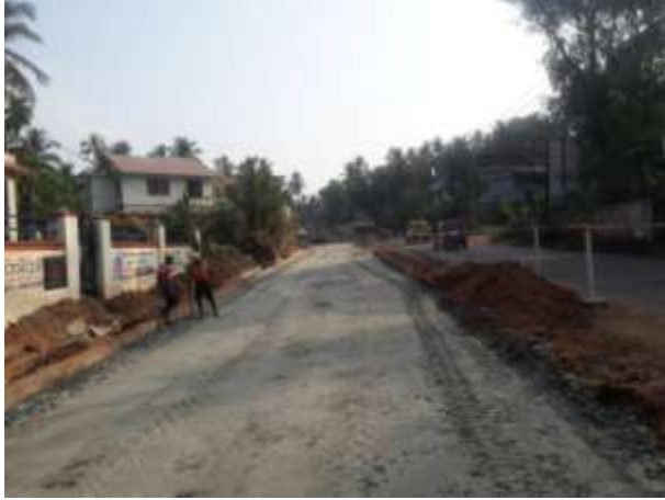
WMM LAYING WORK IN PROGRESS AT KM.4+640 TO 4+800 LHS
