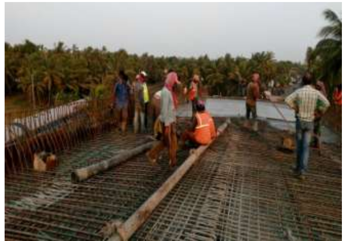
P8-P9 DECK SLAB CONCRETE WORK IN PROGRESS OF THAVAM ROB (KM 7+420)
