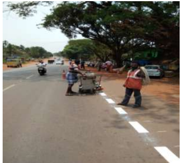
EDGE MARKING IN PROGRESS AT KM 15+350 (LHS)
