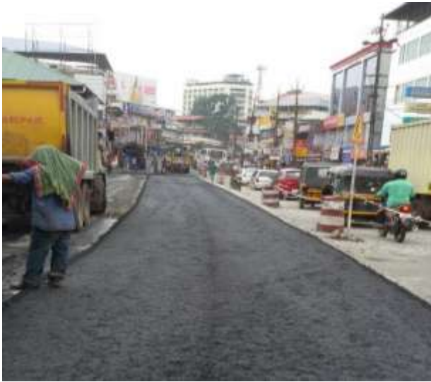
DBM WORK IN PROGRESS AT CH. 16+350 TO 16+550 (LHS)
