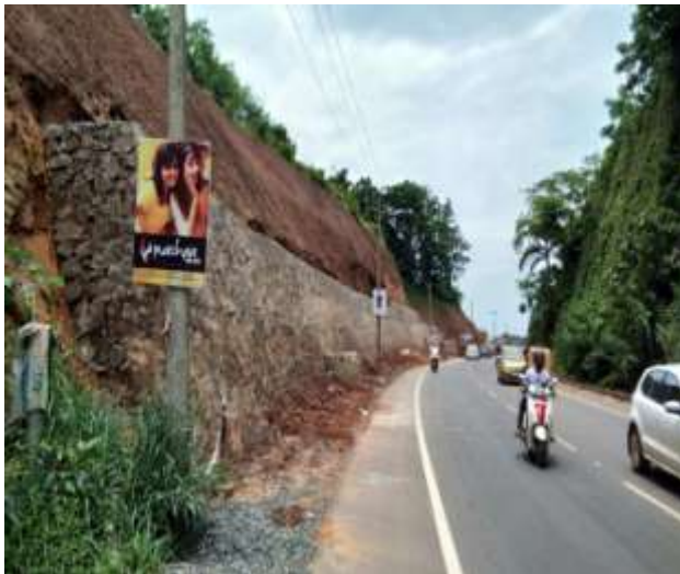
KM: 0+280-405 RHS BREAST WALL WORK IS IN PROGRESS
