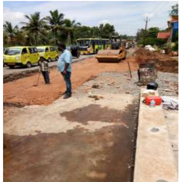
SUBGRADE PREPARATION @ 19+980 TO 20+040(LHS)
