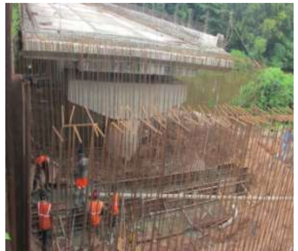
PILE CAP CONCRETING A2 SIDE OF RAMAPURAM BRIDGE (KM 4+260)
