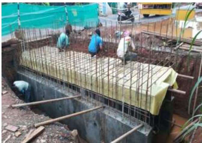
CULVERT SLAB REINFORCEMENT WORK AT 20+746
