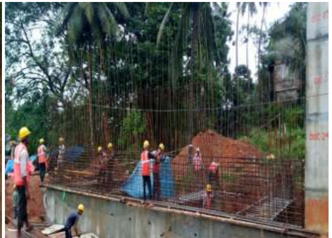
COUNTER FORT RETAINING WALL WORK IN PROGRESS A1 SIDE OF BRIDGE AT KM 42+198
