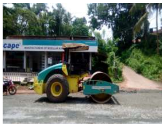
WMM 1 ST LAYER ROLLING AT 9+700
