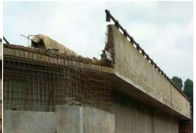
PROVIDING HAND RAIL FOR MINOR BRIDGE CRASH BARRIER (CH: 0+380 KM)
