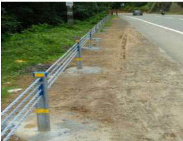
FIXING OF 4 ROPE TYPE WIRE ROPE SAFETY FENCE @ CH : 18+570 TO 18+770 RHS
