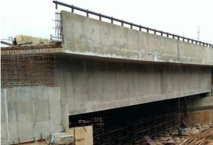
PROVIDING HAND RAIL FOR MINOR BRIDGE CRASH BARRIER (CH: 0+380 KM)
