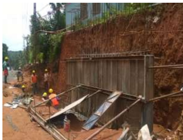
RETAINING WALL CONCRETING WORKS IN PROGRESS AT 4+274
