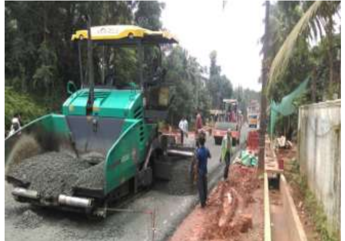
WMM LAYING BETWEEN KM 33+000 TO 34+000
