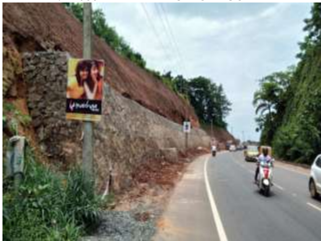
KM: 0+280-405 RHS BREAST WALL WORK IS IN PROGRESS
