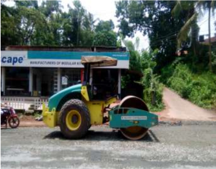
WMM 1 ST LAYER ROLLING AT 9+700
