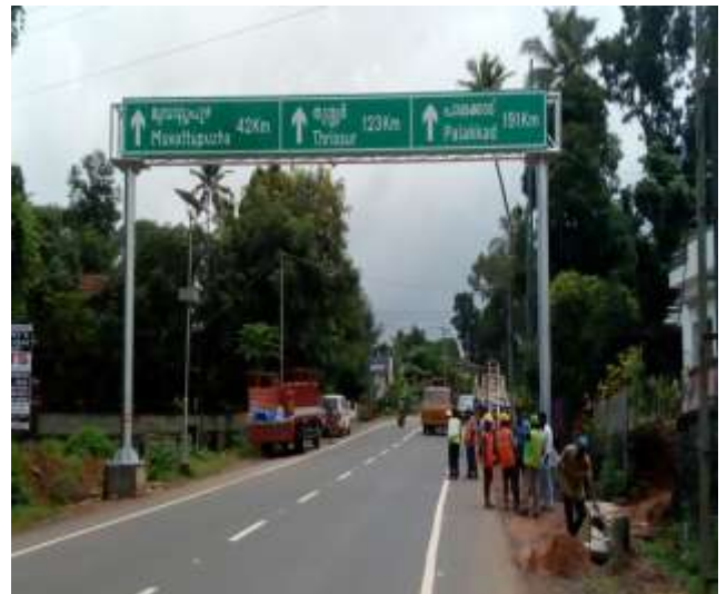
OVER HEAD GANTRY SIGN BOARD @ 0+290KM
