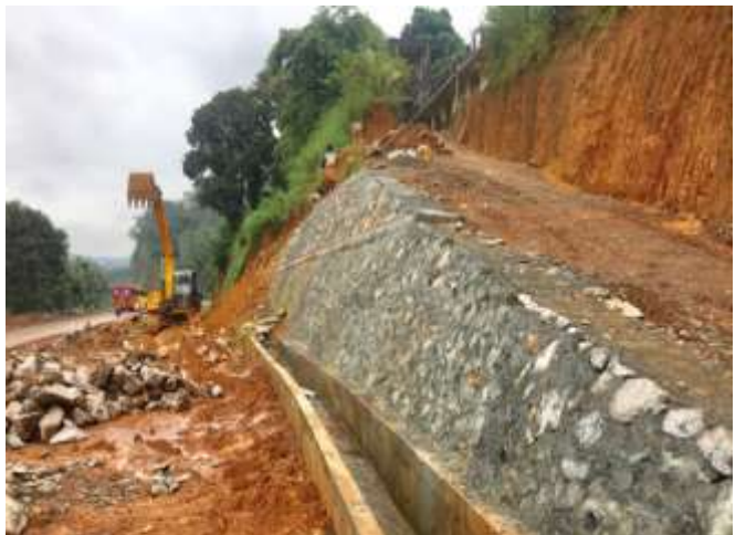
RR MASONRY WALL CONSTRUCTION @ 39+500
