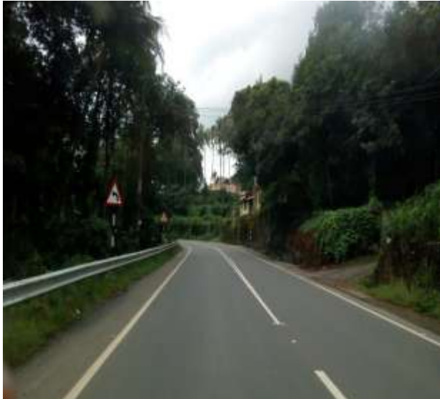
PAVEMENT MARKING & METAL BEAM CRASH BARRIER @ KM 11+450
