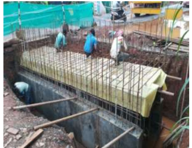
CULVERT SLAB REINFORCEMENT WORK AT 20+746
