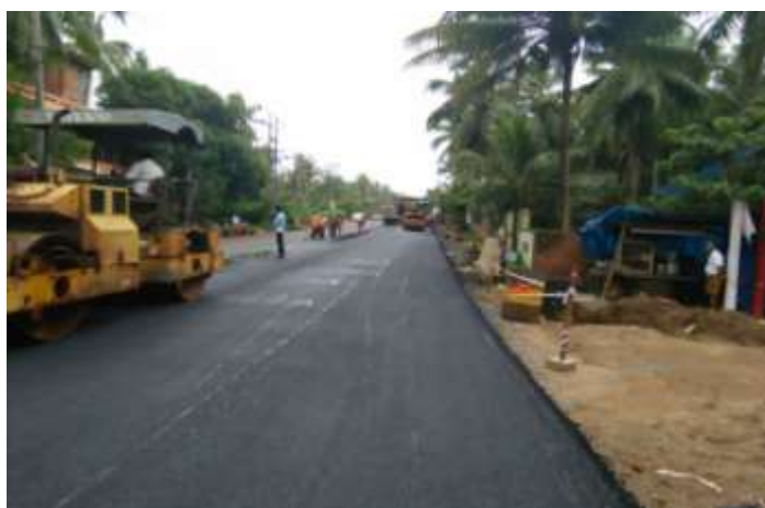
BC LAYING FROM KM 17+250 TO KM 17+450 RHS
