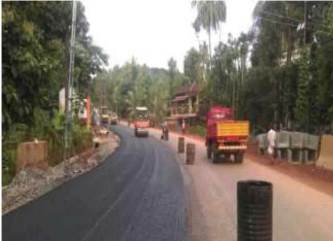
DBM LAYING BETWEEN KM 32+000 TO 33+000
