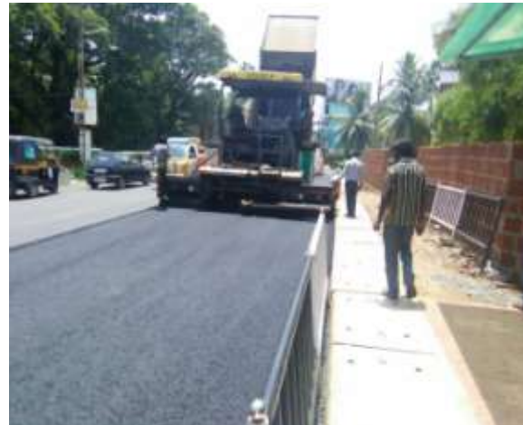
DBM LAYING FROM KM 20+270 TO 20+360 LHS
