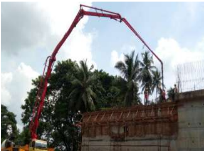
COUNTERFORT RETAINING WALL WORK IN PROGRESS AT 42+198 (A1-IRITY BRIDGE )
