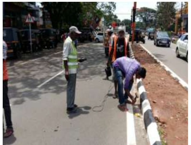
ROAD STUDS FIXING IN PROGRESS KM 10+300 TO 0+600
